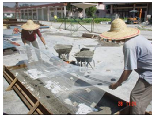
(b) Cast the ferrocement precast layer
