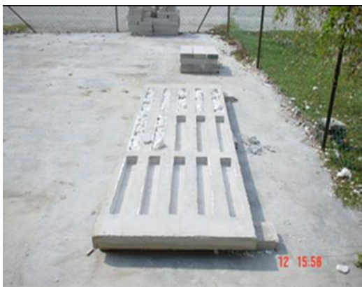
(c) Remove the poliestirè
