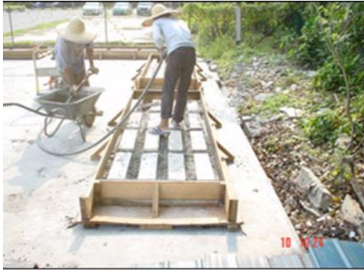
(e) Filling of cast-in situ
