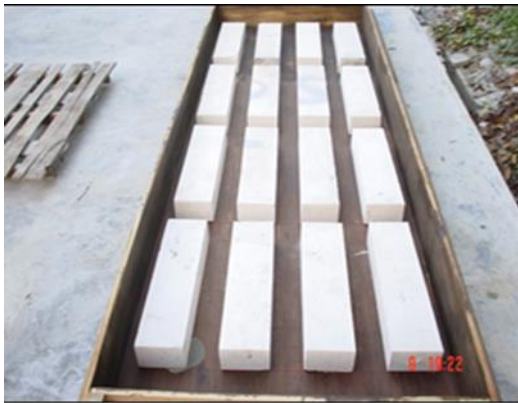
(a) Placed poliestirè in Formwork
